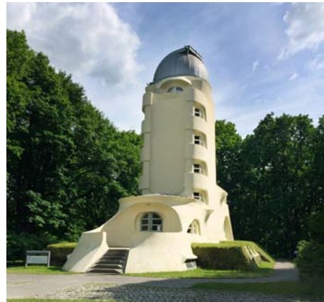
Below: Einstein Tower; Potsdam, Germany; Eric Mendelsohn, 1921-1925 Schocken Department Store; Stuttgart, Germany; Eric Mendelsohn; 1928
