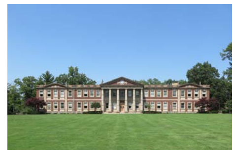
Above: Nela Park Bldg. 308, "Product Management"
