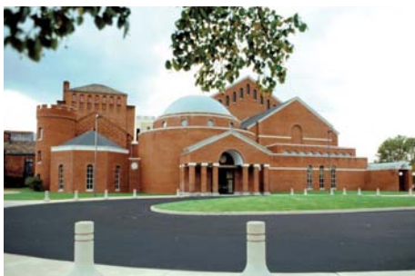
Below: Top: Cleveland Playhouse by Philip Johnson; Demolished by Cleveland Clinic, 2023 Bottom: Cleveland Central Armory, 1393; Lehman & Schmidt; Demolished 1962 for Celebrezze Federal Building
