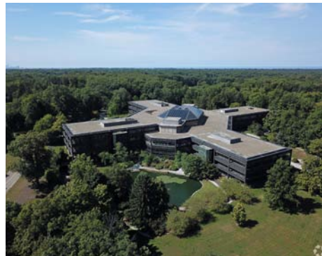
Below: TRW Headquarters before Demolition
